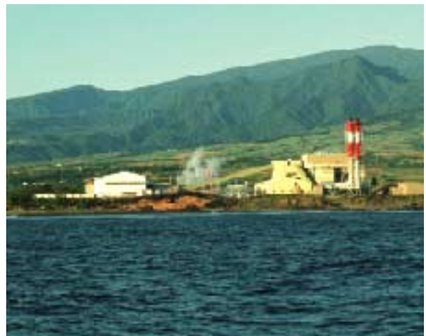
Distillery and power station (Réunion Island)
