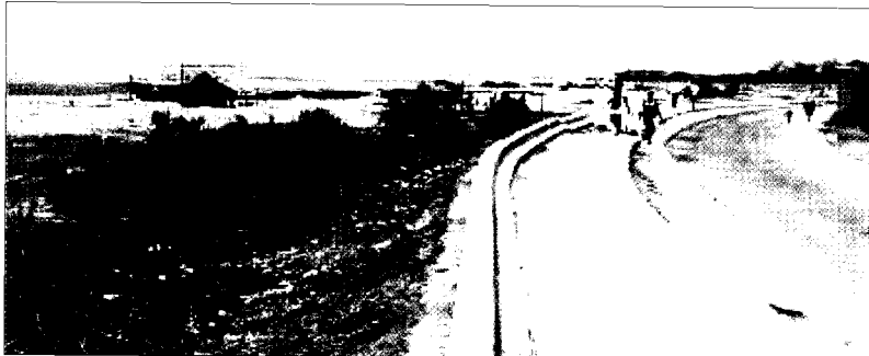
Plate 18: The waterfront at Malindi, Kenya, in 1992, showing the extent of sediment accretion over 30 years
