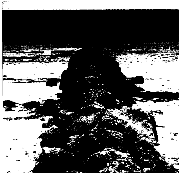
Plate 28: Detail of rock groyne on the Kunduchi shore, north of Dar-es-Salaam, Tanzania
