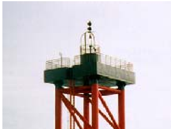
Fig.3 Chuluncho light beacon station
