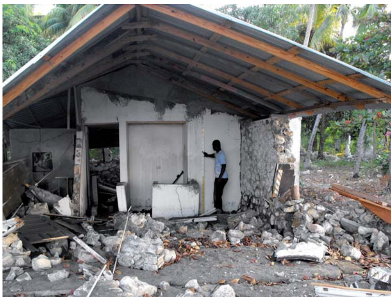
Post-tsunami measurement of run up Haiti following January 2010 event.
