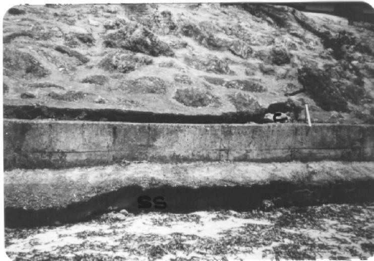
Plate 8 shows seawall along Nyali beach. Note crack (c) on the wall and sediment scour (ss) beneath the wall (September, 1990; Photo by P. Abuodha).
