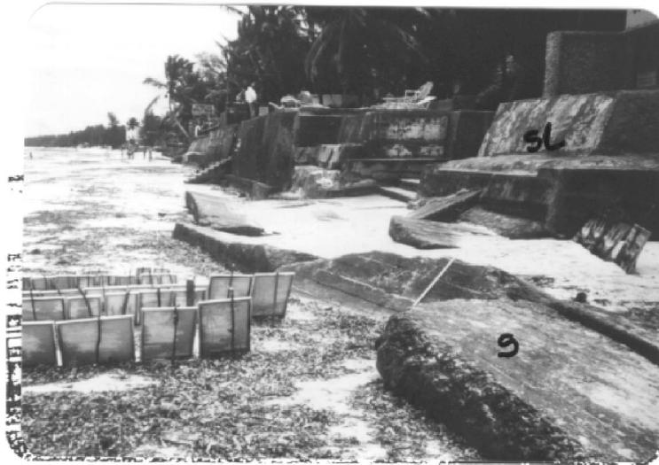
Plate 7 shows a thick seawall (s) at Bamburi. Note another seawall (s1) behind the failed seawall (September, 1990; Photo by P. Abuodha).
