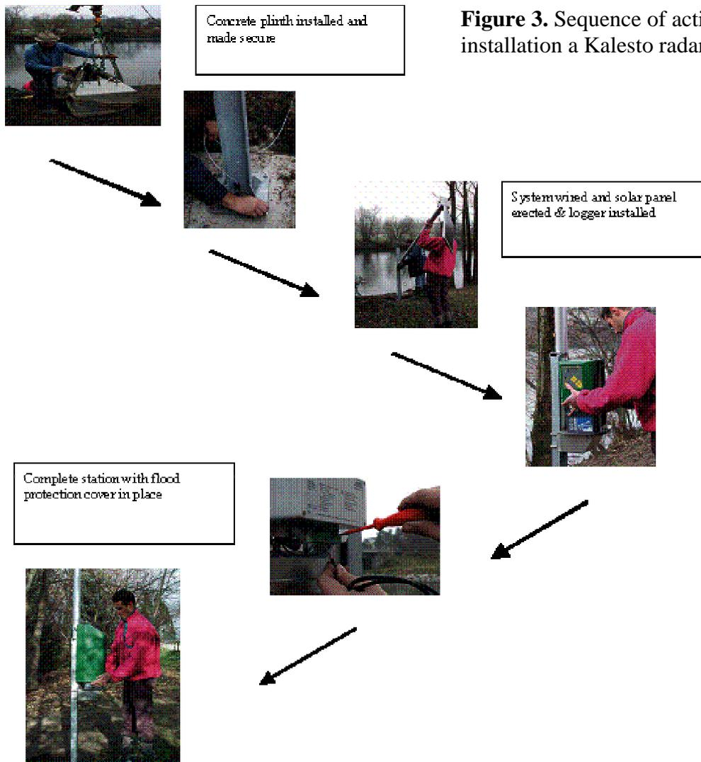
**Figure 3.** Sequence of actions involved in the installation a Kalesto radar gauge.
