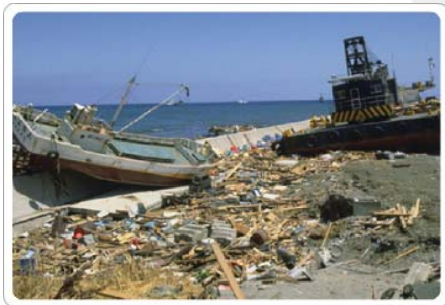
A fishing boat was deposited on top of a concrete shore protection barrier at Aonae, Okushiri Island, Japan during the 1993 Japan Sea tsunami. Note wood debris from houses and other structures scattered about the area. Credit: ITIC
