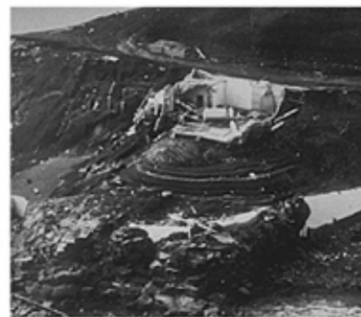
Scotch Cap lighthouse, Unimak, Alaska, before and after a 35-m high tsunami destroyed the 5-story lighthouse on 1 April 1946. The tsunami also caused death and damage in Hawaii, and soon after, the US started its first tsunami warning system.
