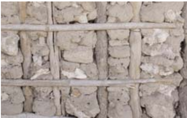
Figure 16 Gastropod shells and coral rubble in house construction in Messano.
