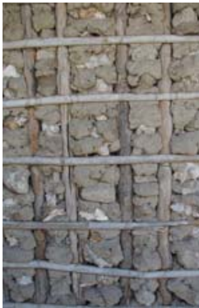
Figure 9 Coral rubble and gastropod shells used in house construction in Northern Mozambique. Source: James Wilson, Kusi Lda
