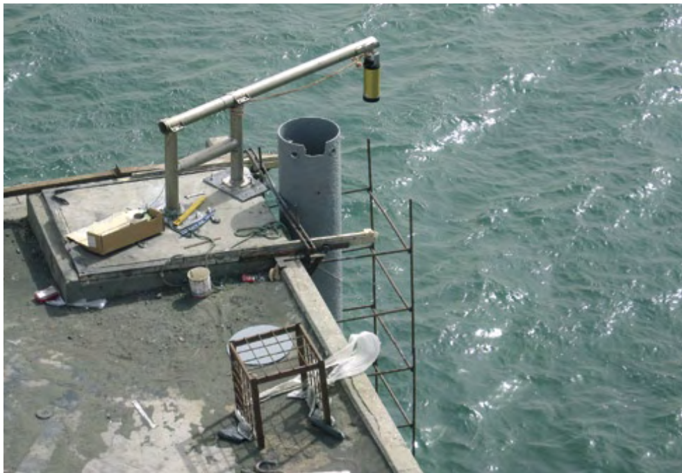
Installation of tide gauge at Nouakchott, Mauritania.
