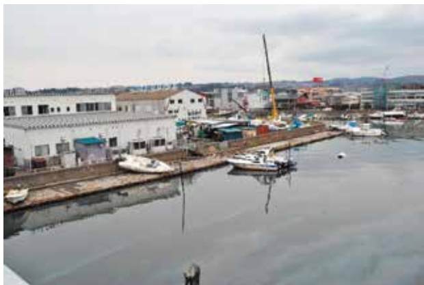
Photo 14. The status of the Teizan Canal in Shiogama city just after the earthquake (taken on March 21, 2011 at the north side of Ipponmatsu Bridge).
