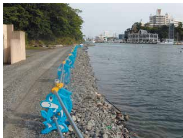
Photo 3. Kesenuma Ko under restoration (taken on May 28, 2016).
