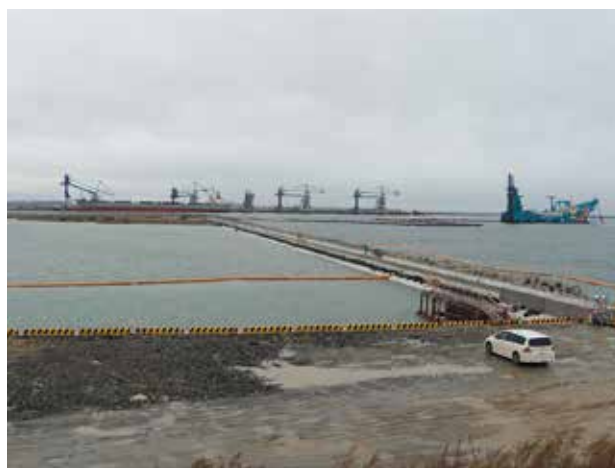
Photo 8. An LNG plant under construction at Soma Ko (taken on November 20, 2015).
