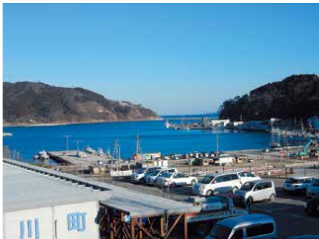
Photo 4. Onagawa Ko under restoration (taken on February 18, 2016).
