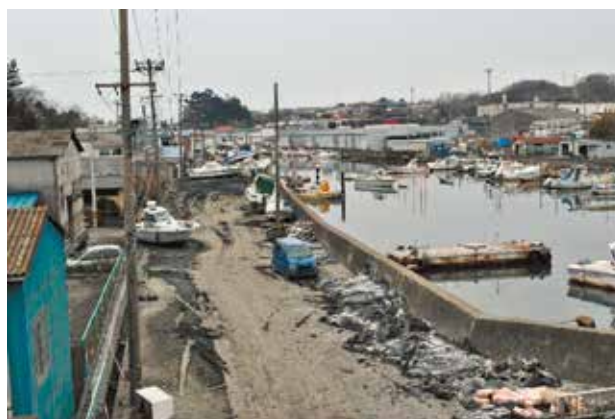
Photo 12. The status of the Teizan Canal in Shiogama city just after the earthquake (taken on March 21, 2011 at the south side of Ipponmatsu Bridge).
