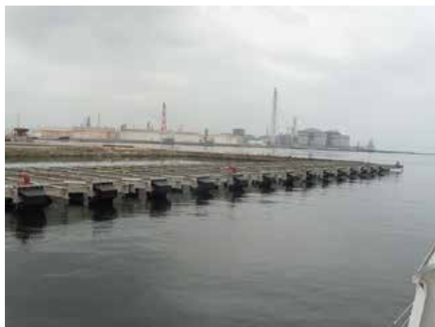
Photo 7. A quay being newly-constructed at Sendai Ko (taken on May 28, 2015).
