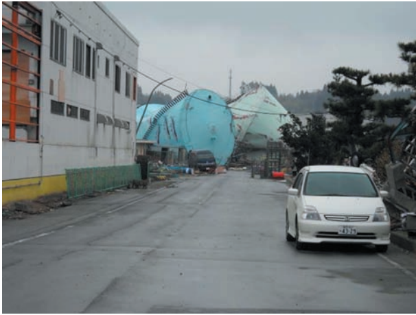
写真7b 倒れたタンク。 Photo 7 b Tanks which fell down.
