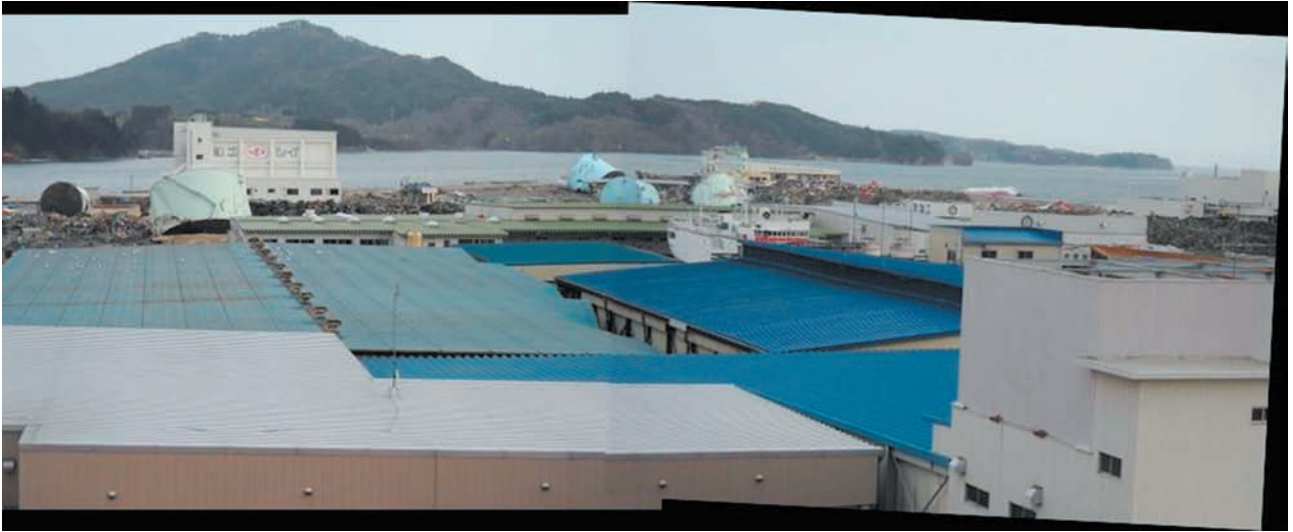
写真7a 気仙沼港石油栈橋。 Photo 7 a Oil pier in Kesen-numa Harbor.
