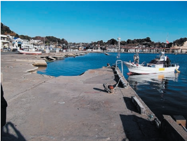
写真 21 c 崩れた防波堤と岸壁 (大津港). Photo 21 c Destroyed breakwater and quay (Otsu Harbor).
